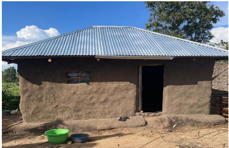
Safer and dignified housing project in Budalangi village constructed through participatory approach
